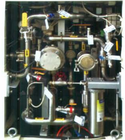
Internal Water Circulation Cooling System
