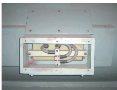
Fig 9 : Typical Alternative Arrangement for Neutral Point Termination
