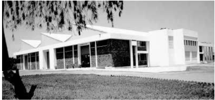
The Ahmednagar factory - manufacturing DC Motors
